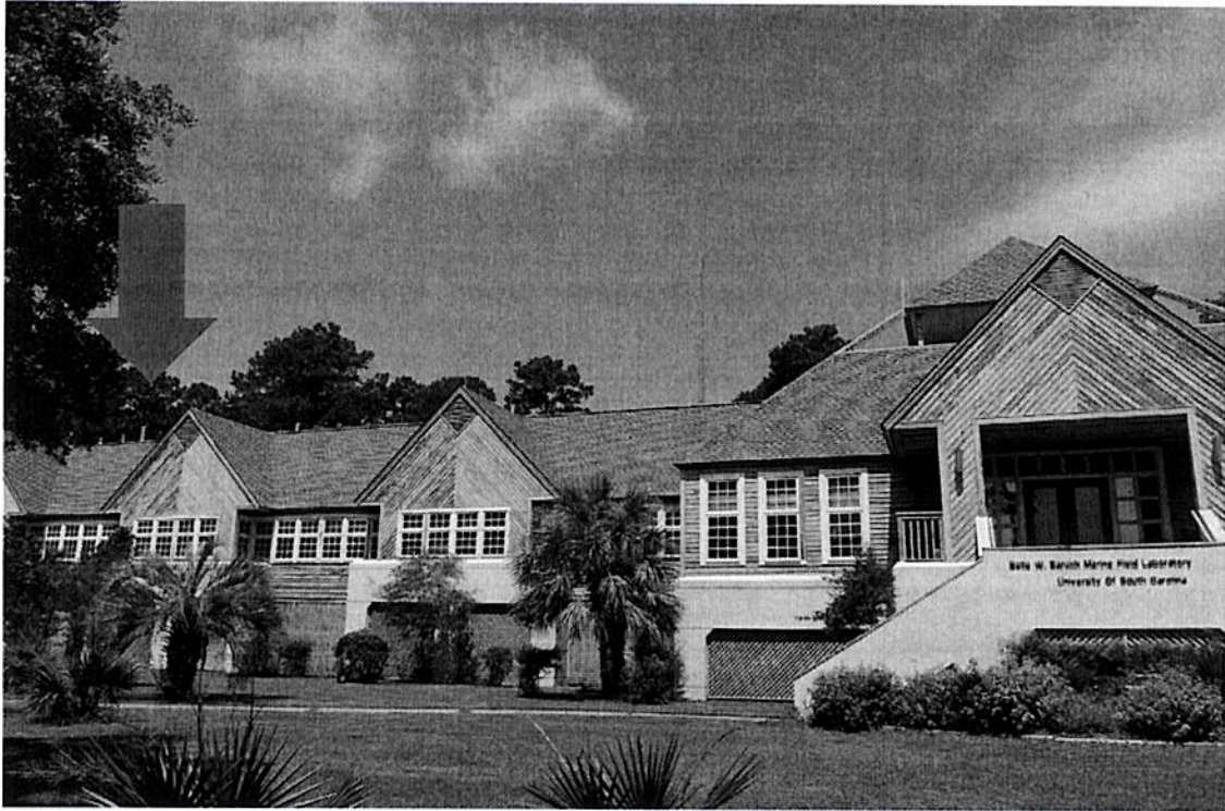
FRONT VIEW OF MARINE RESEARCH FACILITY. RED ARROW SHOWS GENERATOR LOCATION
